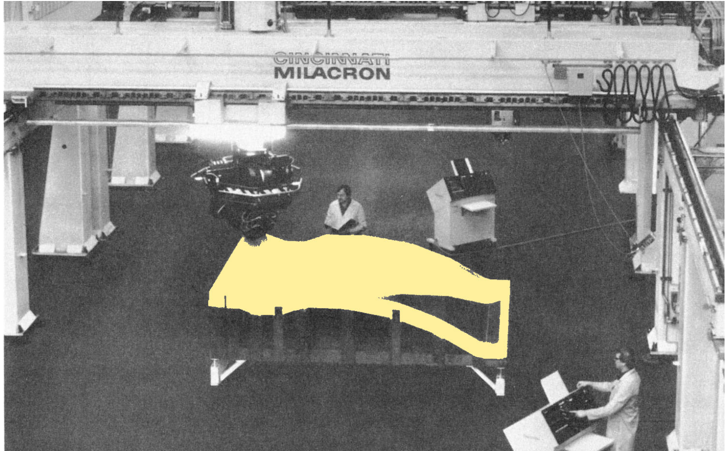
Automated tape-laying machine (photo courtesy of Cincinnati Milacron).
