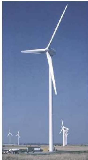
Fig. 1. Horizontal-Axis Large Wind Turbine (Courtesy: GE Energy)
